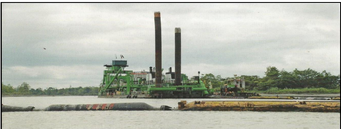
Figure 4.9 Dredges in Operation at Bige
